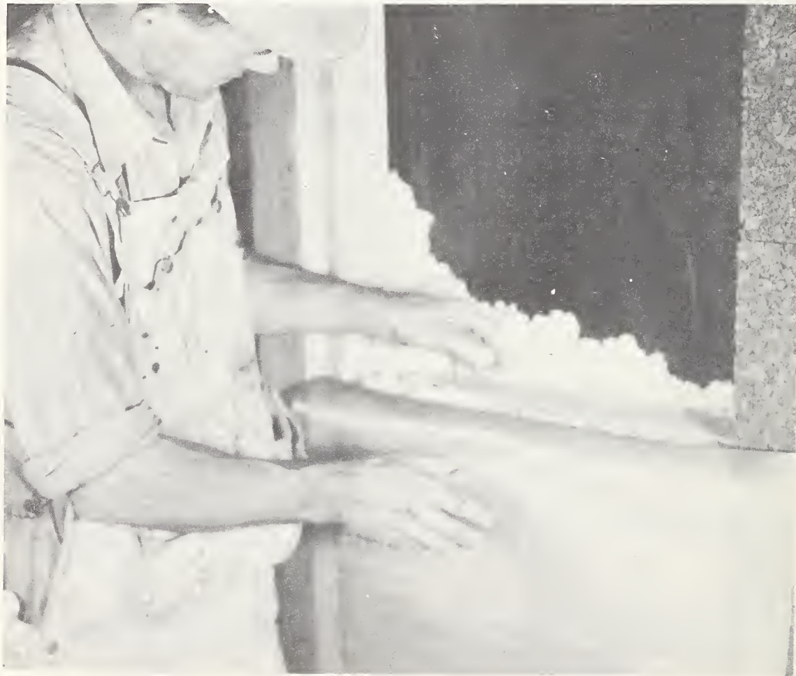
Figure 7.--Placing fill-type insulation in wall.
